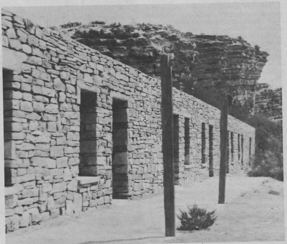
Hot Springs motor court, Big Bend National Park, Texas.
