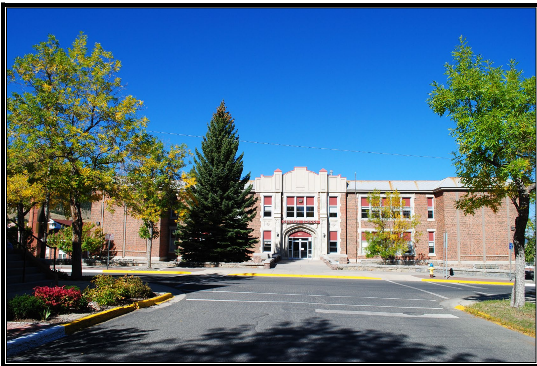
Central School, dated 9/20/2014, before demolition in 2019, photo by Ric Seabrook.
