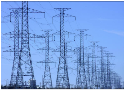
Power facilities and power distribution almost always impact roadways and consequently involve MDT in the permitting and approval process.
