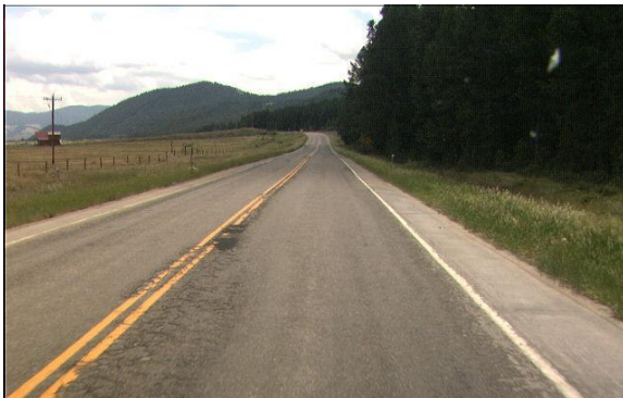
Before: This was Montana Highway 43 in July 2002. The scope of work for the project included reconstructing about 6 miles of roadway and 1.5 miles of overlay.
