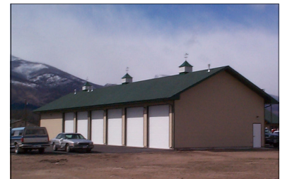
The new bus barn has six bays with room for washing and light maintenance.
