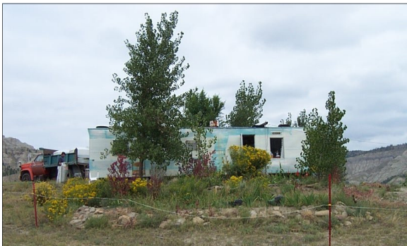
Before: County-owned facilities such as this trailer at McClelland were replaced as part of the upgrade of Montana’s three Missouri River ferries.
