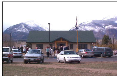
The new Ravalli COA office building also houses offices for BitterRoot Bus.
