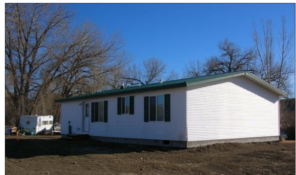
After: This is the new 1,200-square-foot facility at Carter. The buildings at McClelland and Virgelle are similar. All are of modular construction.
