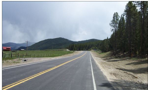
After: This photo was taken in May 2005. A. M. Welles of Norris, Montana, is the primary contractor for the project, which should be completed in July.
