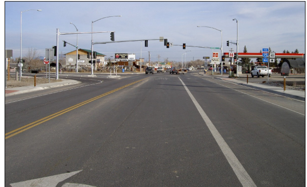
After: This is the same intersection following improvements that included grading and surfacing, sidewalks, water and sewer work, signals, and landscaping. Construction started in April 2004. Blahnik Construction was the primary contractor.
