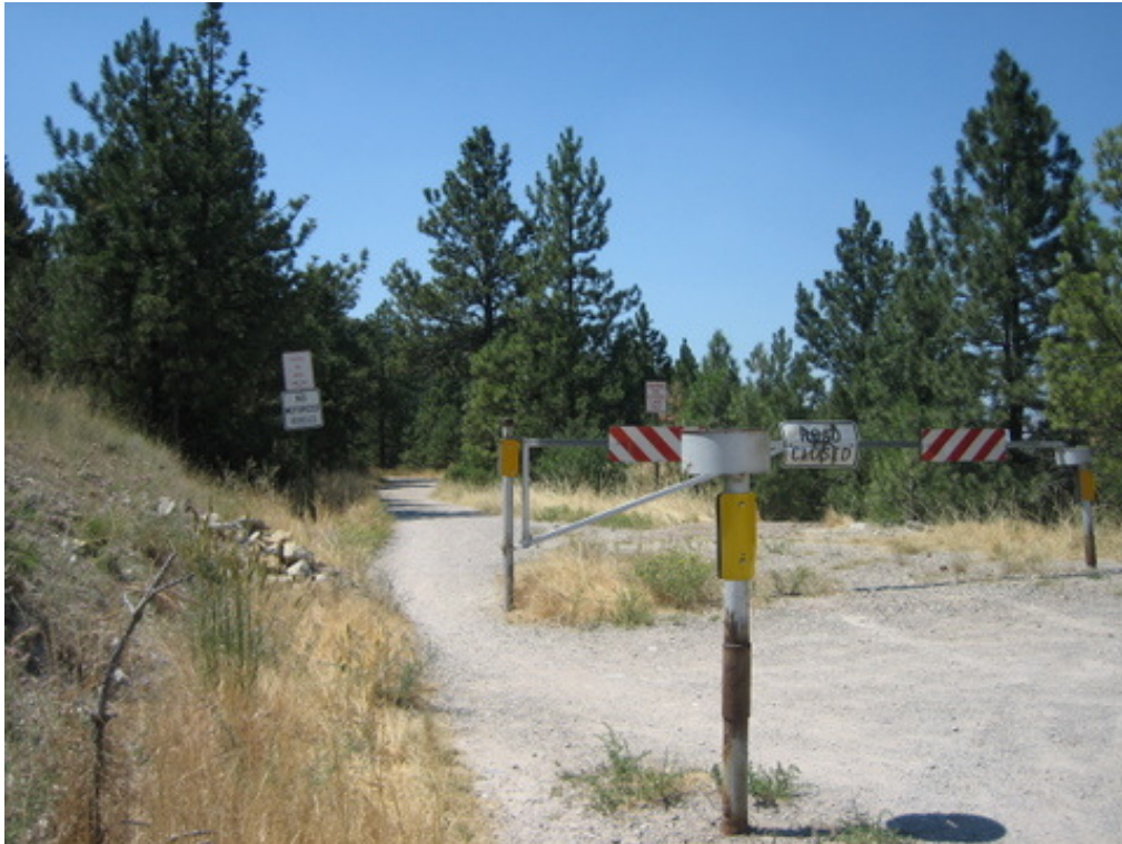
Pedestrian/bicyclist-only segment starting at Boulevard/Silverette St. intersection, west view (2007)
