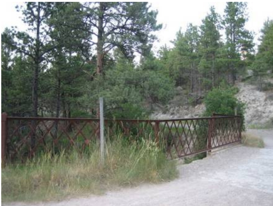
Circa 1910 one-lane lattice bridge on non-vehicular segment (2007)
