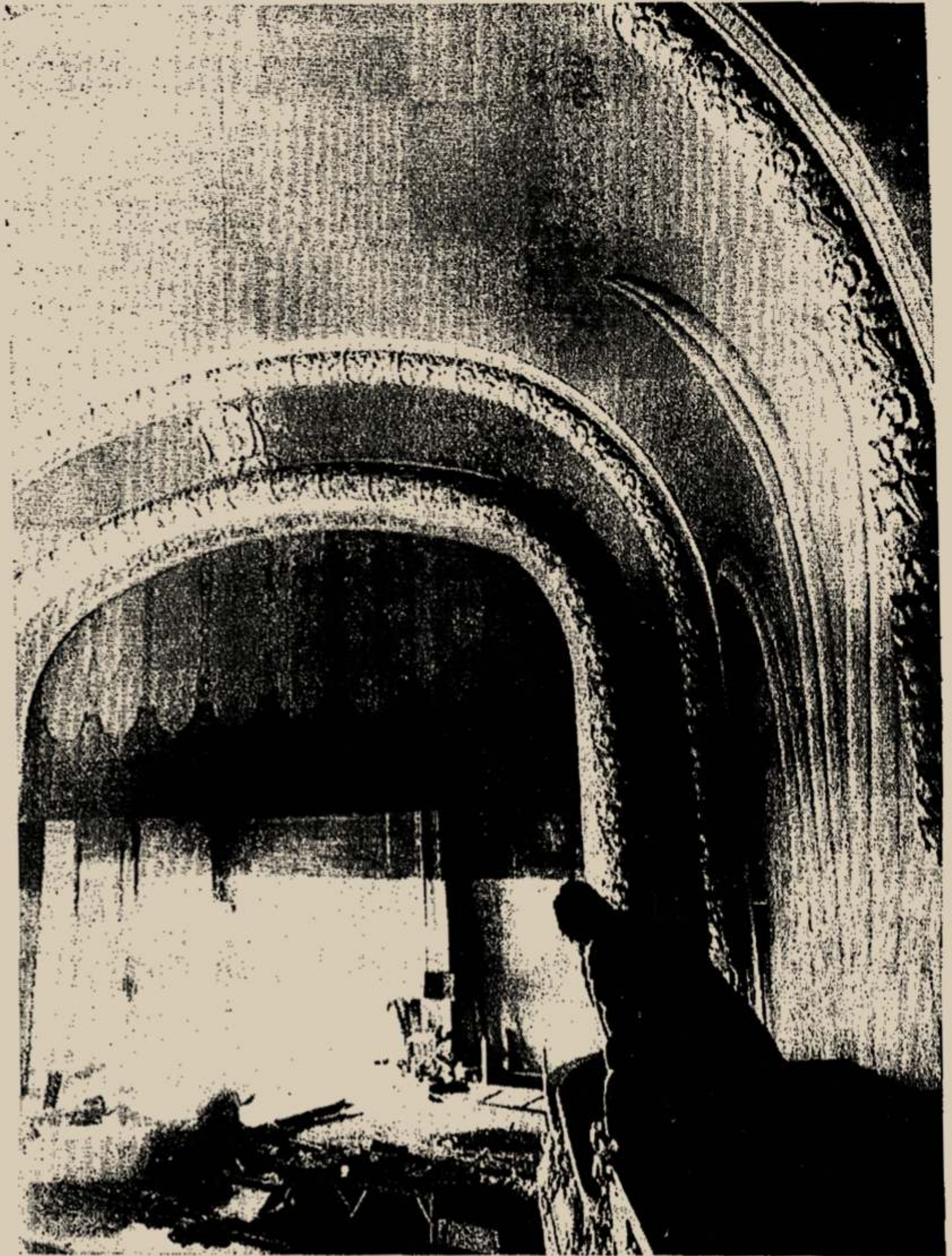
A LAST REGAL LOOK — Charles S. Johnson takes a last look at the interior of the Marlow Theater, not so awestruck now as when the high arches and gargoyles loomed over his five-year-old
