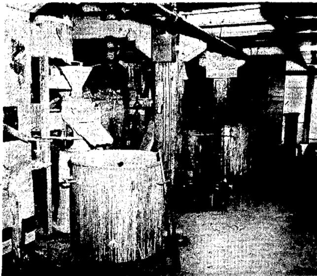
**PAINT IN THE MAKING**—Pigments and oil have been stirred to a heavy paste by the time they are dropped onto the mill floor shown here with Oliver Crowley keeping a careful eye on the processes at the Columbia Paint company manufacturing plant in Helena.
