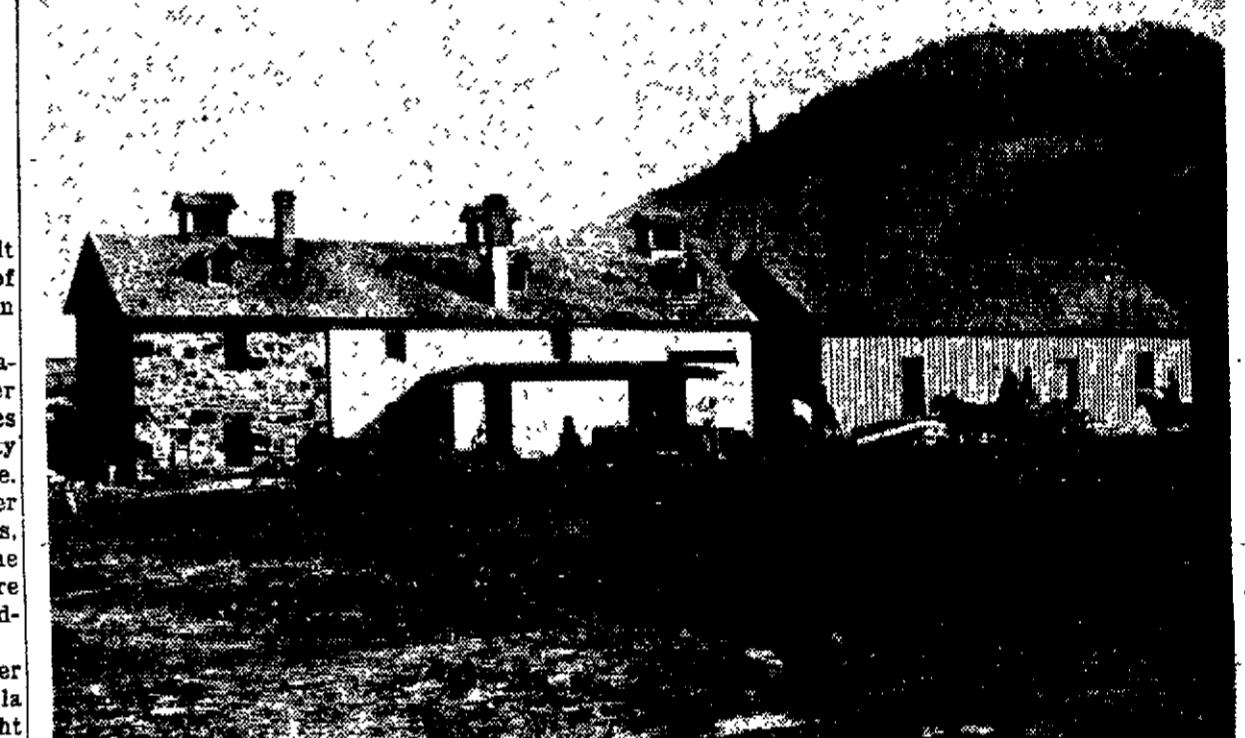
THE ORIGINAL KESSLER BREWERY is shown in this old photograph, believed to be the first taken of the structure. The stone malt house at the left was constructed under the supervision of Charles Beehrer in 1865. Several improvements were added during 1874-85, and the large modern plant of the Kessler rests upon approximately the same site today.
