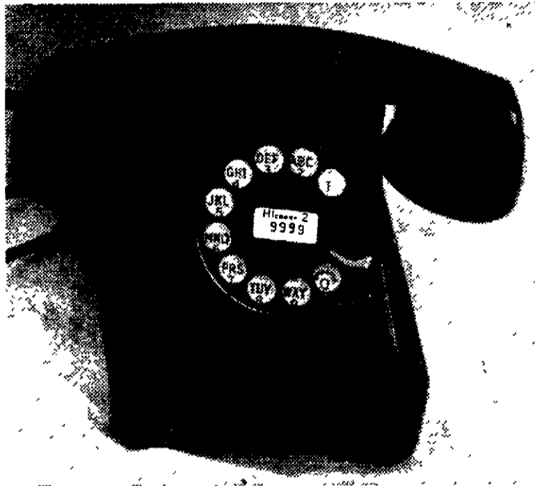
COMPLETED UNIT—A picture of a Helena telephone with the newly installed dial, carrying a sample Hickory 2 number. Although the new dials all have the new numbers when installed, present numbers are left in place over the new number, to be removed by the resident after dial cutover. Telephone users are asked to use the telephones in the usual manner, using the present number, until after conversion. They are warned that the dials cannot be used until that time. At cutover time, the residents can remove the present number and the new dial number will then show.
